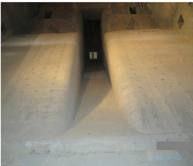
finished shapes are then screwed into place. After fixing any necessary subsequent course of shapes into position, this row of blocks is back-filled with insulating castable material. To protect the metal connection, the hole is sealed off with a ceramic screw.
